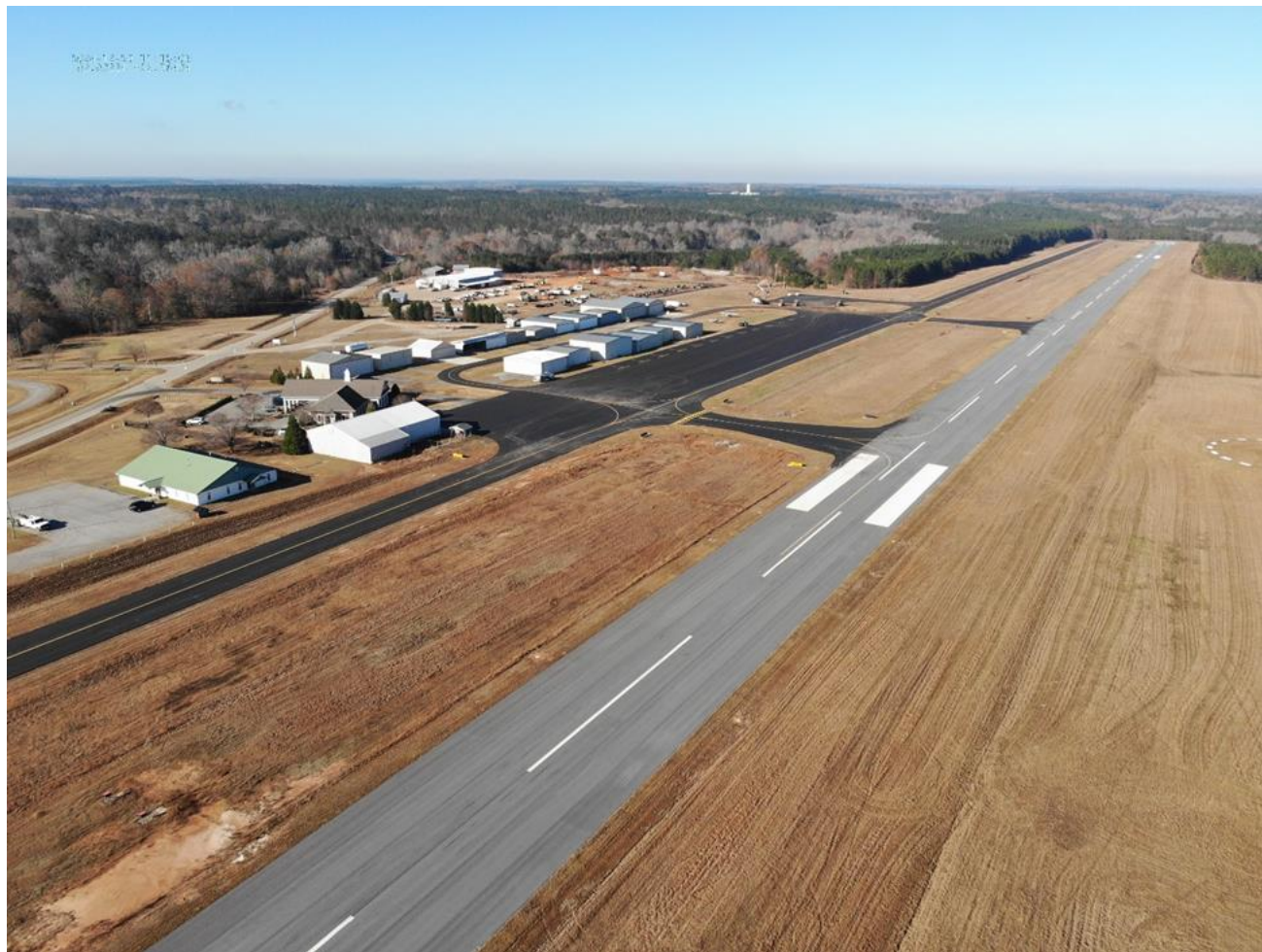
Taxiway after pavement rehabilitation
