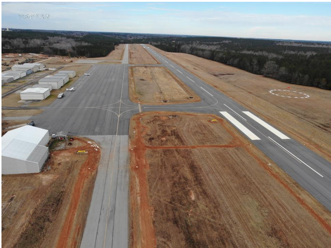
Picture of taxiway prior to construction
